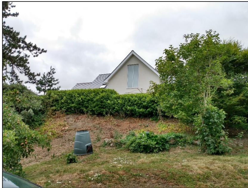
Side bathroom window at Woodpeckers
